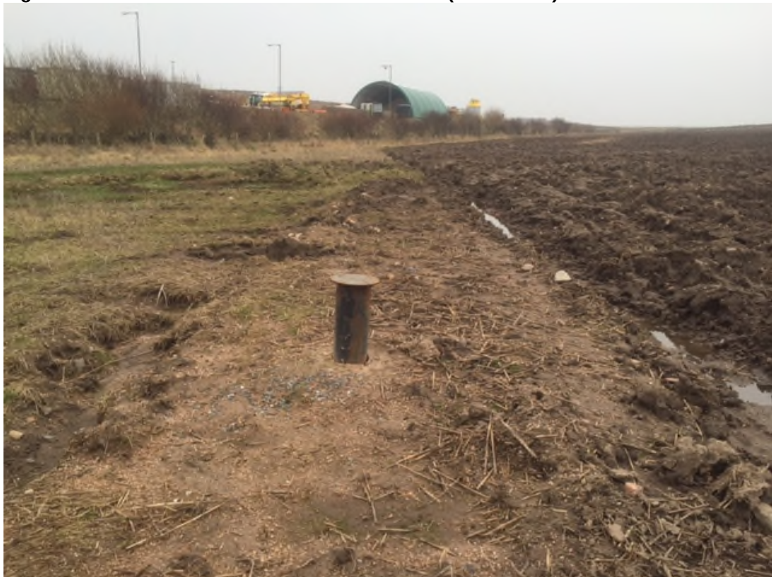
Figure 13.1.1 – Borehole Groundwater Installation (Piezometer)
