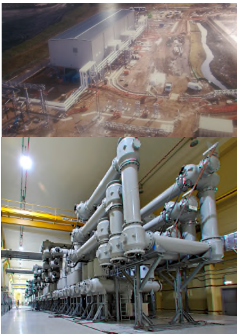
Figure 2.5.1: GIS building, associated GIB and Building Internals
