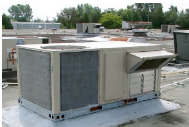
Figure 2.5.5: Air Handling Units (AHU)
