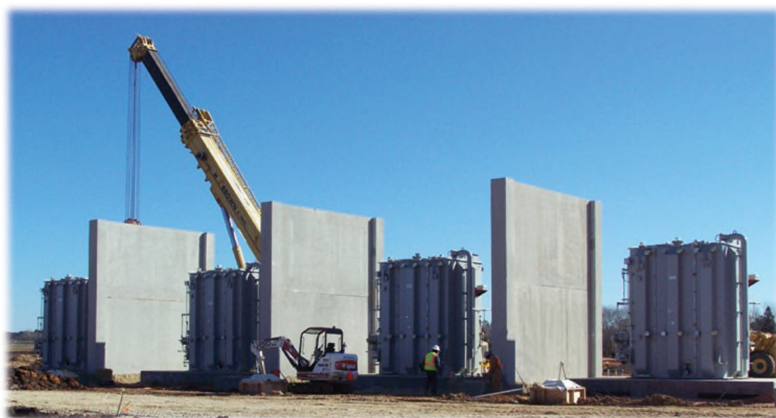
Figure 2.5.4: Super Grid Transformers
