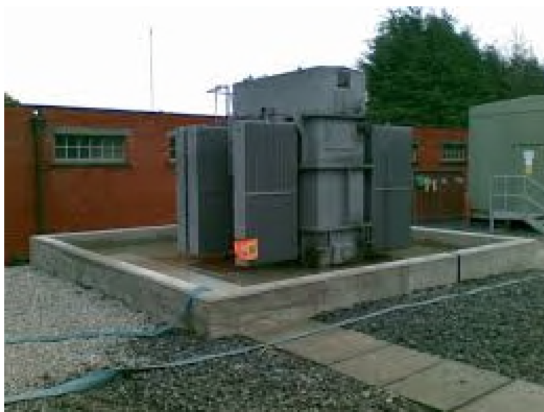
Figure 2.5.3: Auxiliary Transformer
