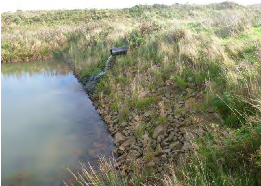
Plate 3: Clearer northern settlement lagoon with rock banks visible, Waterbody 2
